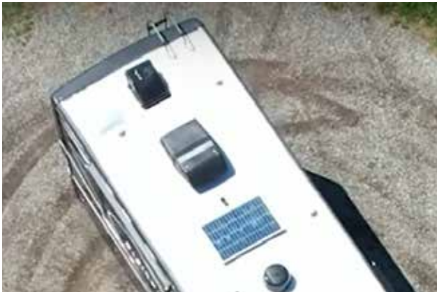
Typical Roof-mounted Solar Panel
