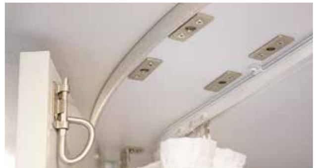
Some bathroom doors provide a second set of door latches, which allows for extra room when in the shower (as illustrated here).
