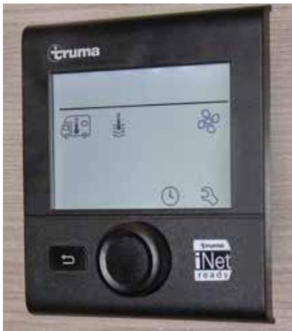
Both the Truma Combi and Aqua-Hot Furnace/Water Heaters are operated by a panel-mounted controller with similar functions and control features. Depending on the floor plan of the motorhome, this control panel is typically mounted on a cabinet or wall surface.
