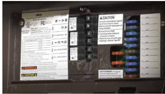
Typical 30-amp circuit breaker and fuse panel. Note circuit and device labels.
