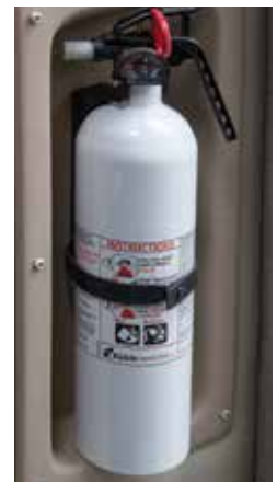
Typical Class B-C fire extinguisher
