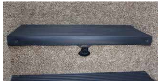
Typical Class C motorhome house battery location (under entrance step)
