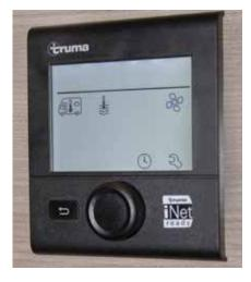
Both the Truma Combi and Aqua-Hot Furnace/Water Heaters are operated by a panel-mounted controller with similar functions and control features. Depending on the floor plan of the motorhome, this control panel is typically mounted on a cabinet or wall surface.
