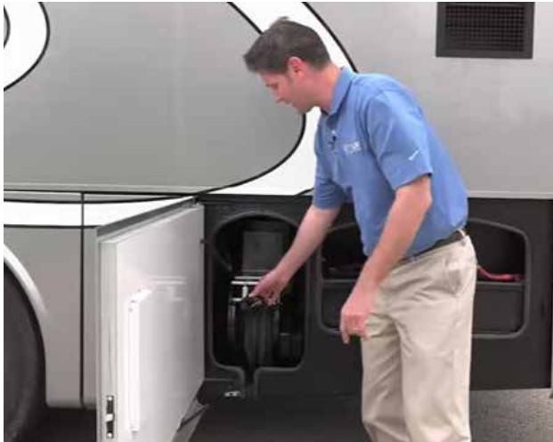
50-amp shore power cord attached to an electrical-powered reel.
