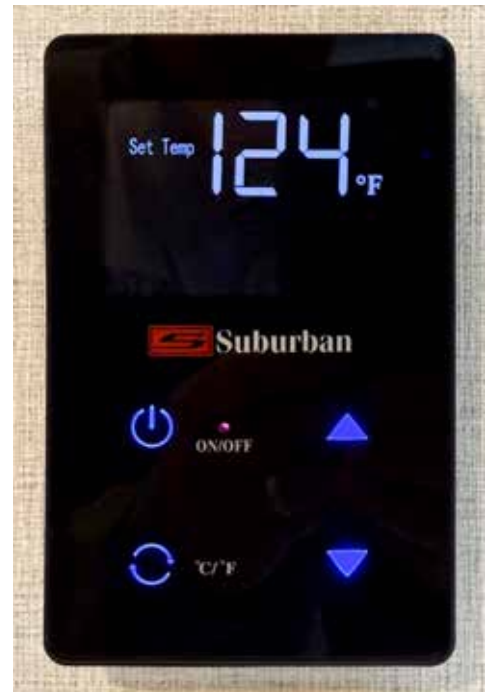
Tankless water heater User Control Panel (UCP) mounted on a bathroom wall
