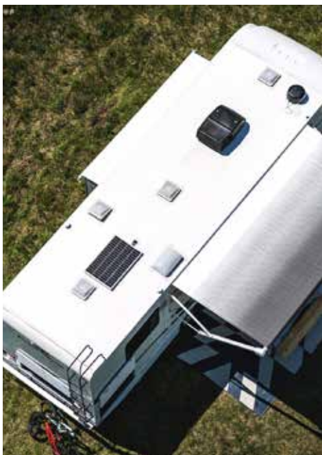
Features installed on an RV's roof require maintenance attention.
