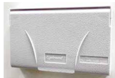
Typical exterior GFCI-protected 120 volt AC outlet.
