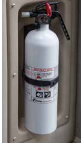
Typical Class B-C fire extinguisher
