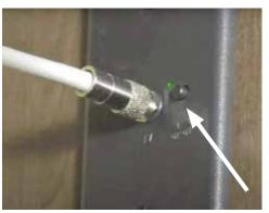
Antenna/Cable push-button selection switch with green LED
