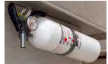
Typical Class B-C fire extinguisher
